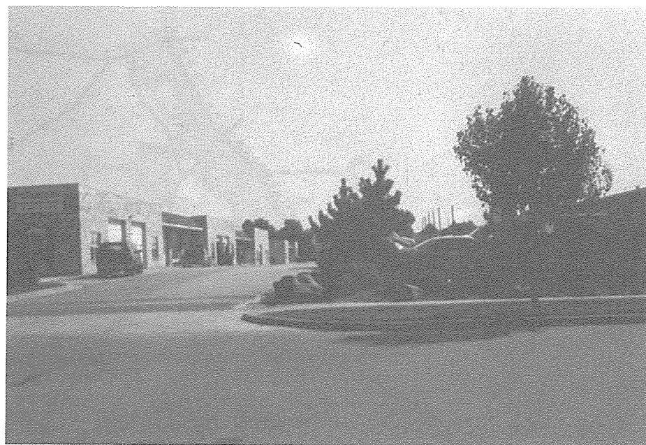
Light industrial, warehouse, office and quasi-public uses occupy 1.1 million square feet in the Penn-Belt and Randall Industrial Parks, located southeast of the MD 4/Beltway interchange.
