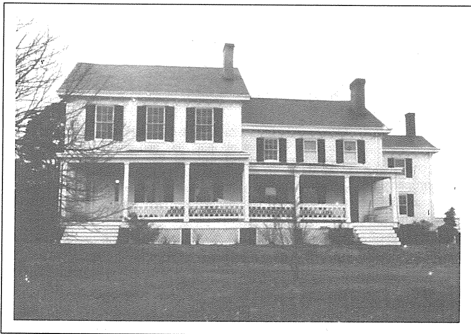
The Cottage, an outstanding example of architectural telescoping, was constructed in 1846 for Charles Clagett and later enlarged. It is located at the Chesapeake Bay Foundation's Clagett Center north of Old Marlboro Pike.
